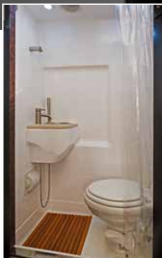
Two-piece fiberglass shower with porcelain toilet, solid surface sink
